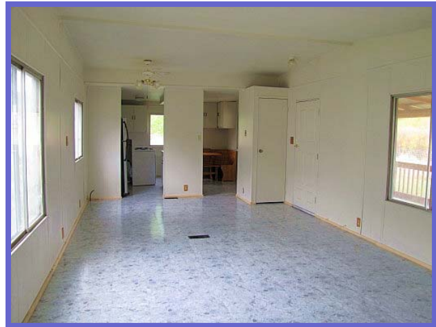
Clean and nice, the living room features new linoleum!
