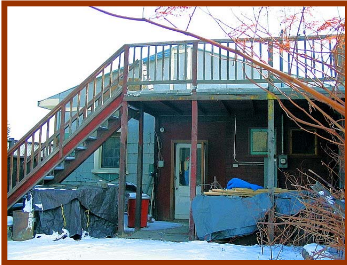
View of the back of building. Stairwell leads to unfinished loft area.
